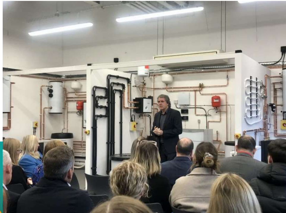
Nov 2024 opening of the Heat Pump facility at City of Liverpool College
